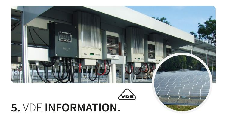
In accordance with installation regulation IEC 60364-5-52 (DIN VDE 0100-522.3), cable systems must be designed in such a way that damage caused by the ingress of water is avoided in all cases.
